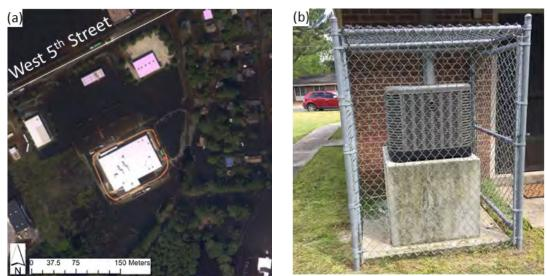
Figure 2-10. Examples of visible individual-level mitigation efforts in Lumberton implemented before the 2018 Flood; (a) Temporary perimeter flood protection around international retailer building (NOAA 2018); (b) Elevated air conditioning condensers in a public housing complex.
